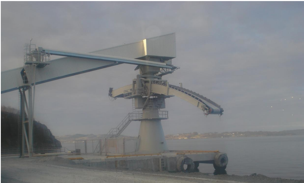
Figure 9.7: Picture of discharger, land-side cargo handling equipment
