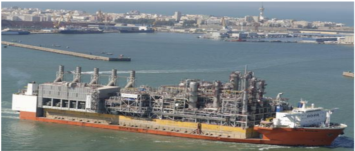
Figure 10: THE SNØHVIT LNG PLANT ON THE BARGE “BLUE MARLIN”.
