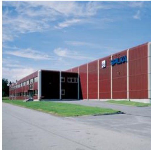
Picture 3 Spilka's marketing and production facility in Ålesund (Spilka, 2011c)
