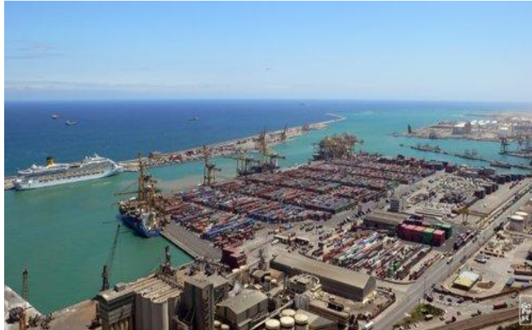
Figure 3.10) Port logistics activity zones: Barcelona Port logistics centers (Sophie, 2007)
