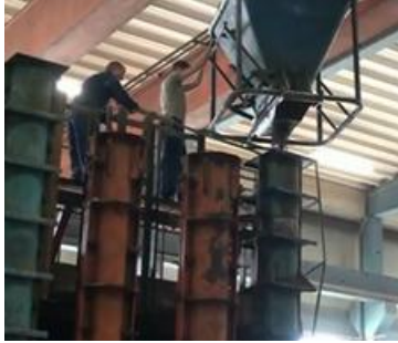
Picture 5 Pouring concrete into a dies when producing beams
