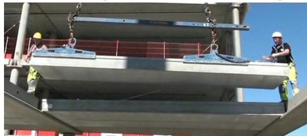
Picture 6 Assembling hollow core elements at a building site
