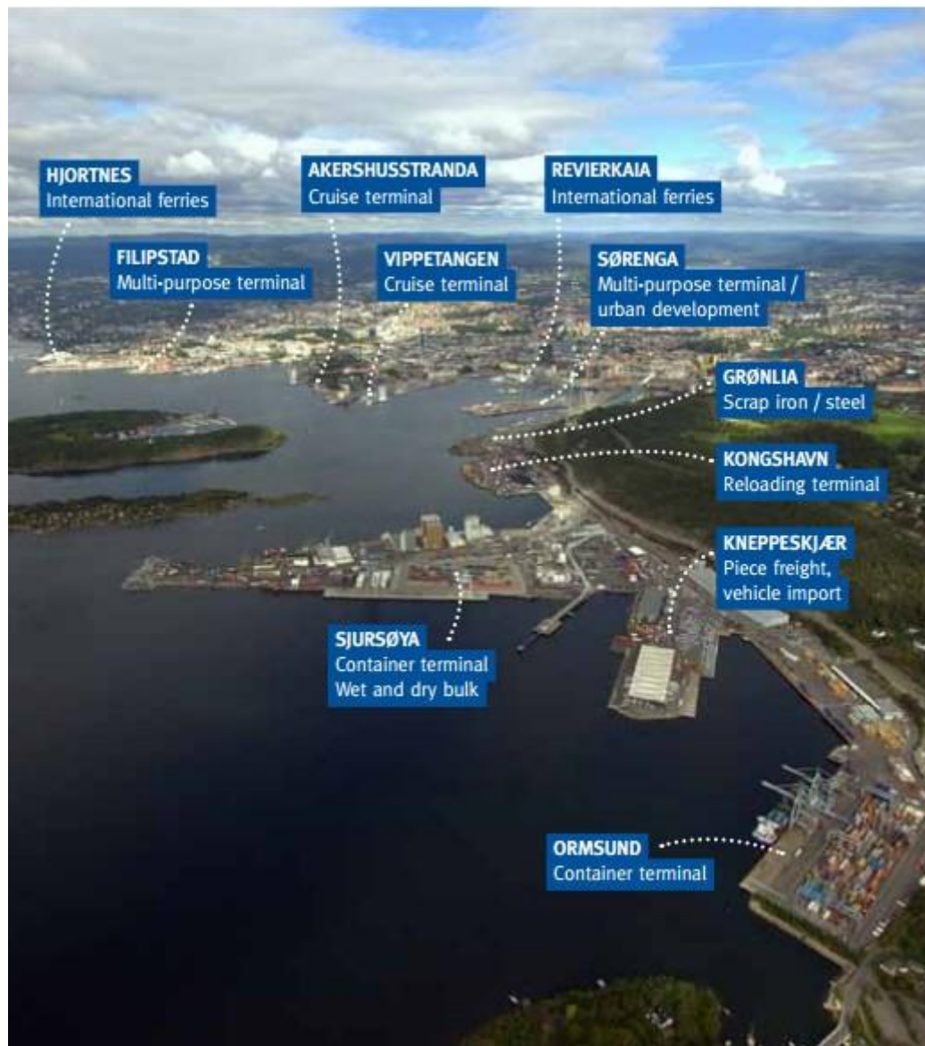
Figure 5.1: Bird's-eye view of port of Oslo
