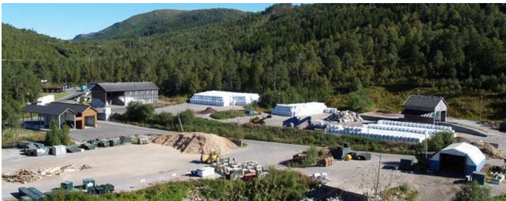
Figure 3: RIR plant (RIRwebpage)
