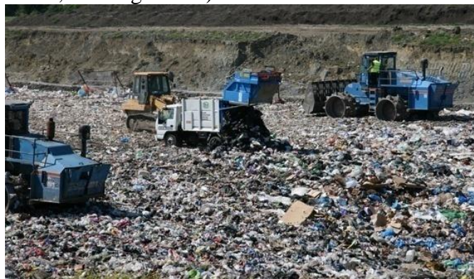
Figure 11: A typical landfill in Great Britain (SmartPlanet 2008)
