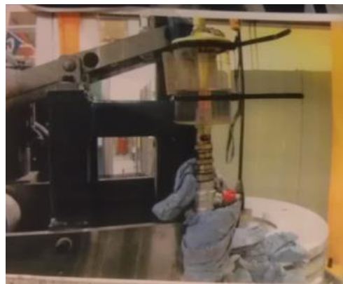
Figure 4.6: The Leakage of Oil near PL5 machinery and its primary solution
