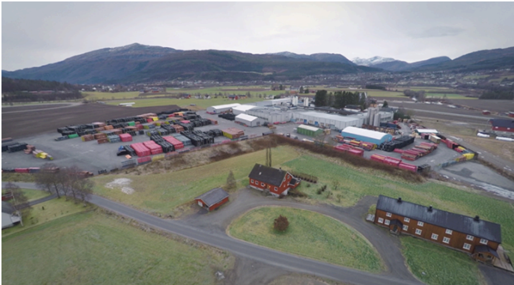
Figure 12: Pipelife AS (Surnadal, Norway)
