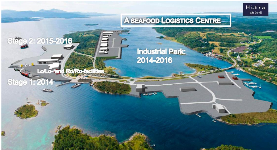
Picture 3.5. Hitra and Industrial park (Hitra kommune 2016)
