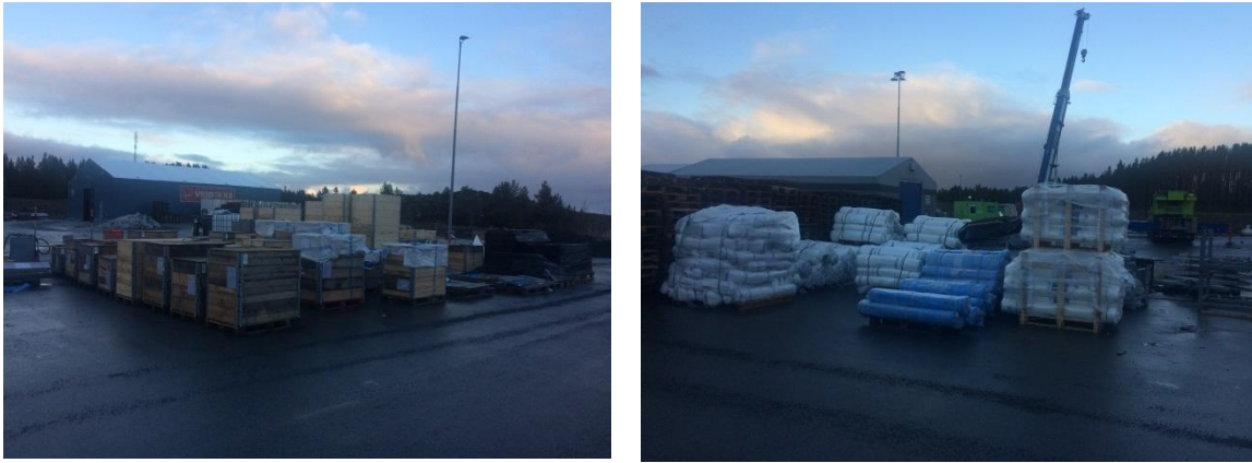
Figure 19: Hall 6 – outside; Storage of pyrogel and monarflex (bulk material)
