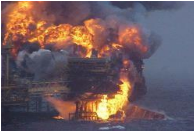
Figure 1 Mumbai High North (MHN) complex after vessel collision
