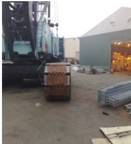
Picture: Truck obstacles at the shipyard
