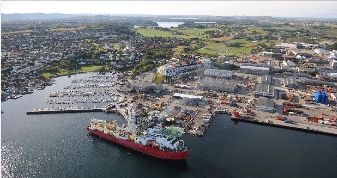
Figure 2.5: The onshore supply base
