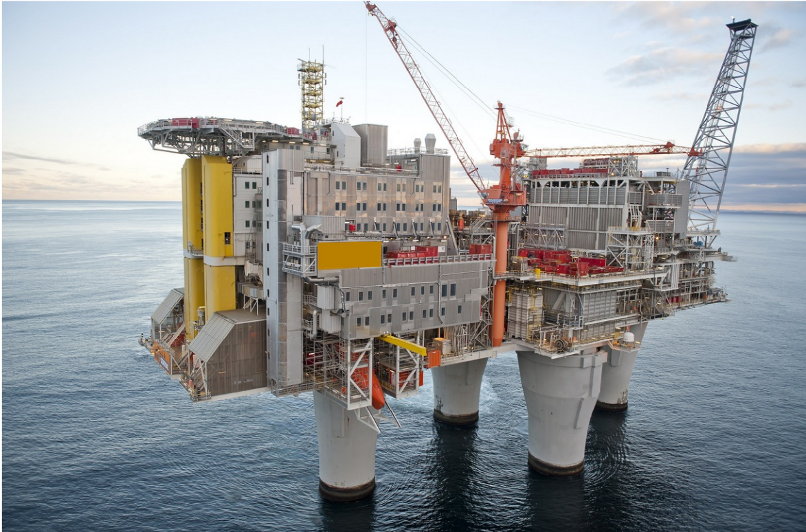
Figure 2.2: Offshore oil production platform, one of the subtypes of the conventional fixed platform
