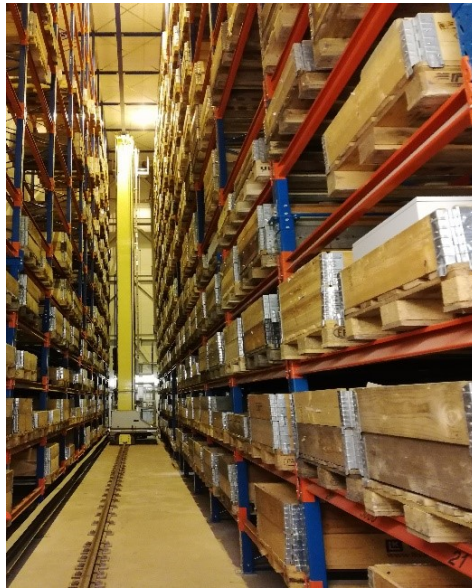
Figure 18: The shipyards automatic pallet storage (AS/RS)
