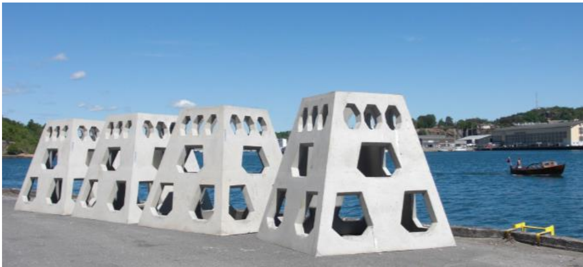
Figure 7: Artificial reef for large fish (adopted from Aagaard (2010, p. 26))
