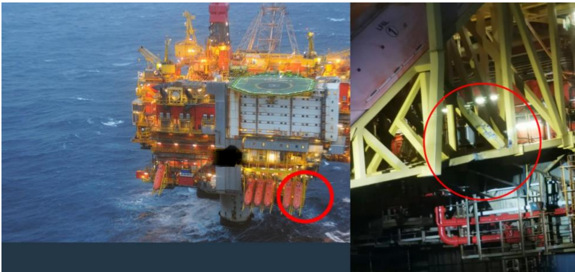
Figure 4: Picture of the damage at Platform A . Foto by: NTB scanpix
